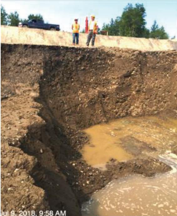
Picture 6 - Conditioned soil densification - First stage
