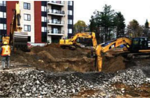
Picture 5 - Exposed steep excavation face in earlier conditioned soil
